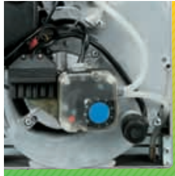
Air pressure switch
